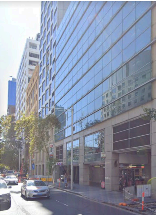
Photo of existing colonnade at Sussex Street
