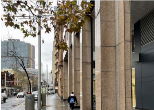
Existing Colonnade at 140 Sussex Street
