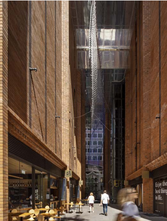
161 Clarence Street - Existing Through Site Link
