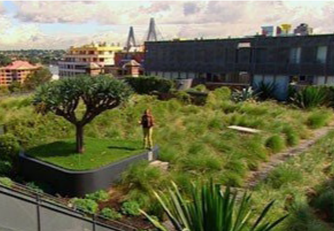
/ Rooftop Garden Spaces
